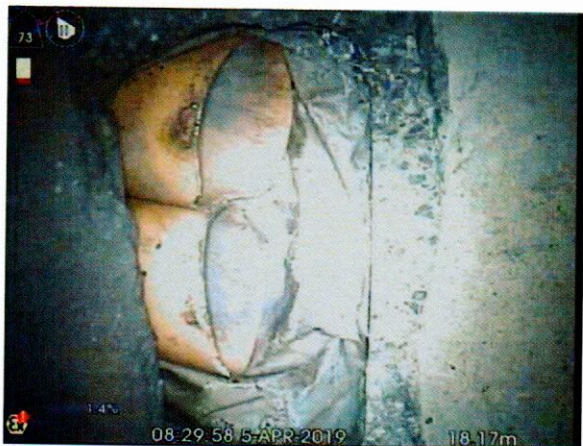
S6X_bdf240ab-03ce-4839-a13b-4a7ff26210f2_20190405_092 906_364.jpg, 00:02:43, 18.17 m Connection other than junction at 12 o'clock, diameter:
