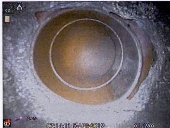
S4X_0a9403e3-fb40-4f72-b1bf-ef6ebd8fc1bf_20190405_081320_079.jpg, 00:08:11, 61.19 m Connection other than junction at 12 o'clock, diameter:
