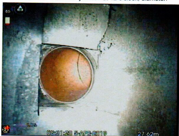
S6X_d6038f54-fdae-433f-a67f-0de6ba9aa6ba_20190405_093 028_351.jpg, 00:03:47, 27.62 m Connection other than junction at 12 o'clock, diameter:
