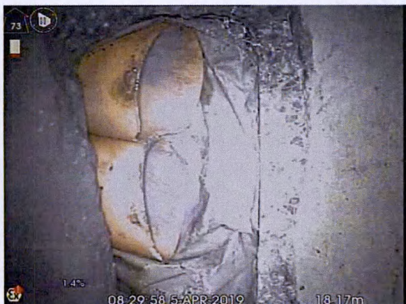
S6X_bdf240ab-03ce-4839-a13b-4a7ff26210f2_20190405_092 906_364.jpg, 00:02:43, 18.17 m Connection other than junction at 12 o'clock, diameter:
