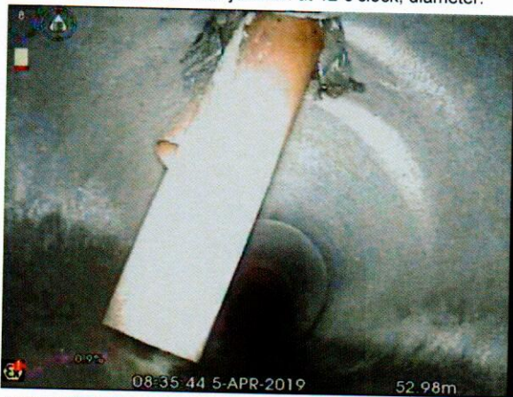
S6X_884f3d3d-f874-4854-8418-3b70886c52c6_20190405_093453_196.jpg, 00:07:02, 52.98 m Connection intruding at 12 o'clock, diameter: 100mm,
