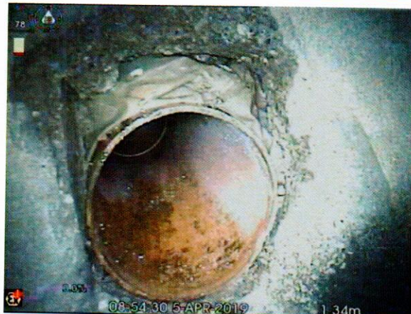
S7X_5389aa5f-4fe3-4cf8-b377-cfb7861908ba_20190405_095 338_868.jpg, 00:01:38, 1.34 m Connection other than junction at 12 o'clock, diameter:
