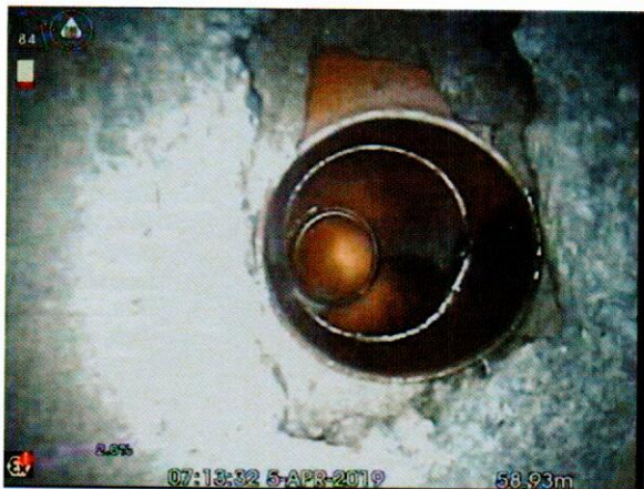
S4X_0e1e6e37-3caa-43e9-b2cf-042f1139d628_20190405_081240_534.jpg, 00:07:39, 58.93 m Connection other than junction at 12 o'clock, diameter:
