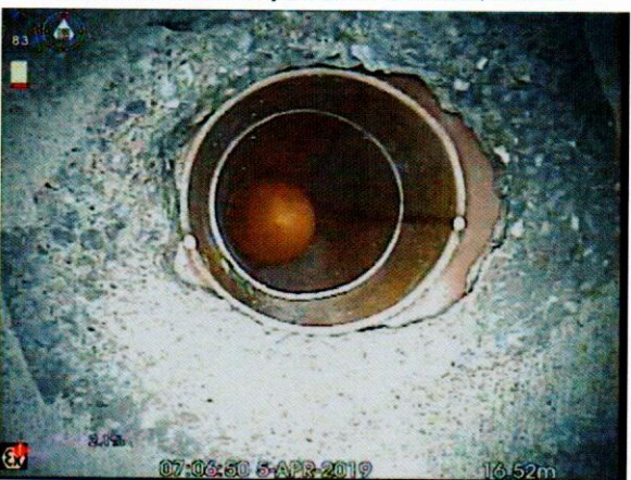
S4X_0a309ee2-7cfd-4233-bd52-868781fad4a2_20190405_080558_786.jpg, 00:02:01, 16.53 m Connection other than junction at 12 o'clock, diameter:
