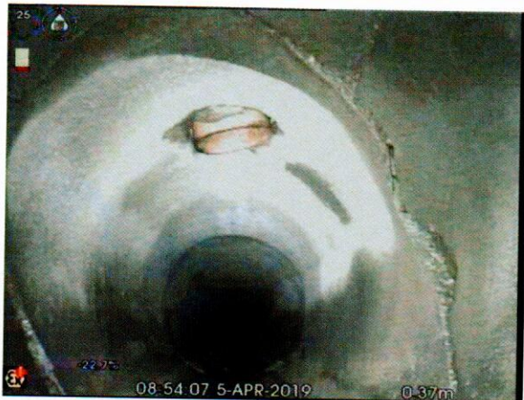
S7X_7668e268-54dd-4054-bff4-0173f5f9763b_20190405_095 314_961.jpg, 00:01:21, 0.37 m Cracks, spiral from 12 o'clock to 12 o'clock
