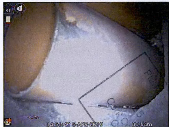
S11X_b51732fa-f87c-498b-98f5-c59dd0c10ad3_20190405_155550_998.jpg, 00:03:25, 30.64 m Connection other than junction at 1 o'clock, diameter: 150mm
