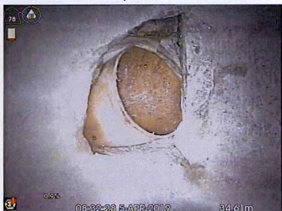
S6X_ddbe4989-b184-447f-9b4f-07cca075102e_20190405_09 3136_478.jpg, 00:04:39, 34.61 m Connection other than junction at 12 o'clock, diameter:
