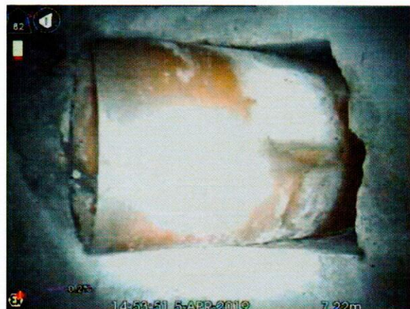
S11X_8c26414c-5570-4c5c-9c45-72a3d62b1144_20190405_155300_478.jpg, 00:00:53, 7.22 m Connection other than junction at 1 o'clock, diameter: 150mm
