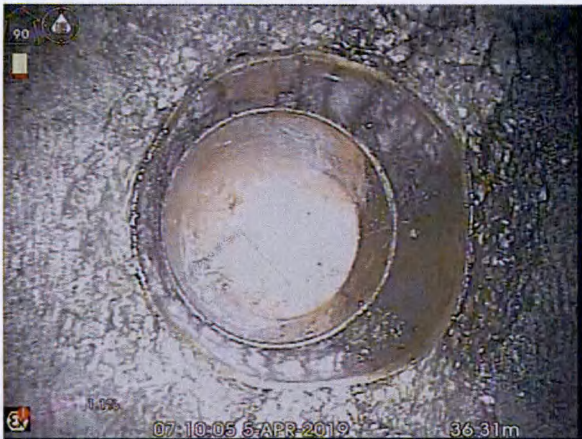
S4X_8113a11a-517e-4edd-8ac4-bde4a3698e20_20190405_080913_677.jpg, 00:04:43, 36.31 m Connection other than junction at 12 o'clock, diameter:
