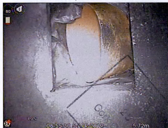
S7X_ff2f0039-0154-4204-b1e9-e659e7926ade_20190405_095439_124.jpg, 00:02:16, 5.72 m Connection other than junction at 1 o'clock, diameter: 100mm
