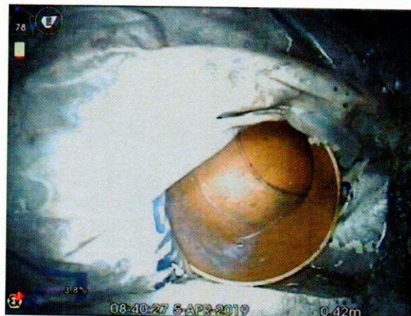
S5X_03b0457f-bb8e-468f-9713-1786b92e3fda_20190405_093935_556.jpg, 00:00:14, 0.42 m Connection other than junction at 2 o'clock, diameter: 100mm
