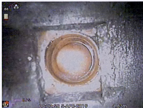
S5X_693240fd-ed56-427d-b066-fe6b68a06725_20190405_090306_660.jpg, 00:00:30, 4.83 m Connection other than junction at 12 o'clock, diameter:
