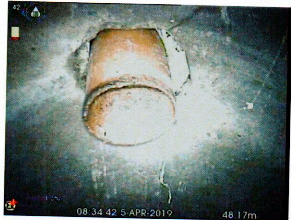
S6X_0d19f72f-ee95-4bcb-a8f3-93b19fae9762_20190405_093350_333.jpg, 00:06:23, 48.17 m Connection intruding at 12 o'clock, diameter: 100mm,
