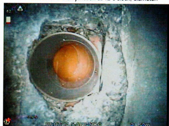
S5X_4b0726a5-1b8e-4719-8026-5574e0baccf4_20190405_090622_341.jpg, 00:03:30, 21.52 m Connection other than junction at 12 o'clock, diameter:
