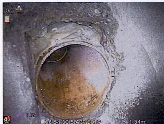
S7X_5389aa5f-4fe3-4cf8-b377-cfb7861908ba_20190405_095338_868.jpg, 00:01:38, 1.34 m Connection other than junction at 12 o'clock, diameter:
