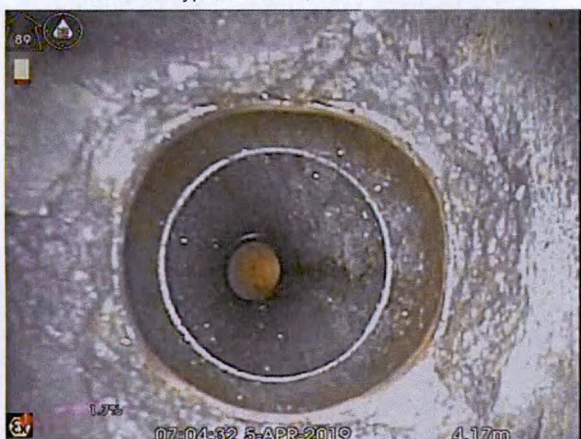
S4X_6021ae2c-959a-4f2c-99e0-d2c84a075fe2_20190405_08 0341_009.jpg, 00:00:38, 4.16 m Connection other than junction at 12 o'clock, diameter:
