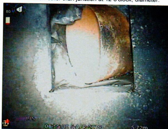
S7X_ff2f0039-0154-4204-b1e9-e659e7926ade_20190405_095 5439_124.jpg, 00:02:16, 5.72 m Connection other than junction at 1 o'clock, diameter: 100mm
