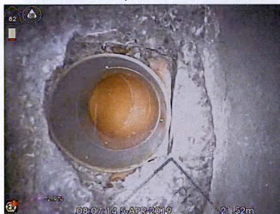
S5X_4b0726a5-1b8e-4719-8026-5574e0baccf4_20190405_090622_341.jpg, 00:03:30, 21.52 m Connection other than junction at 12 o'clock, diameter:
