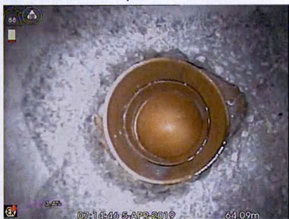
S4X_a38e43f0-4d8b-475b-90dc-9483a57644e7_20190405_081355_262.jpg, 00:08:39, 64.09 m Connection other than junction at 12 o'clock, diameter:
