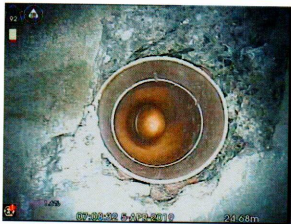
S4X_f6729a63-531b-46b9-9aaf-873fb425f930_20190405_080740_702.jpg, 00:03:25, 24.68 m Connection other than junction at 12 o'clock, diameter:
