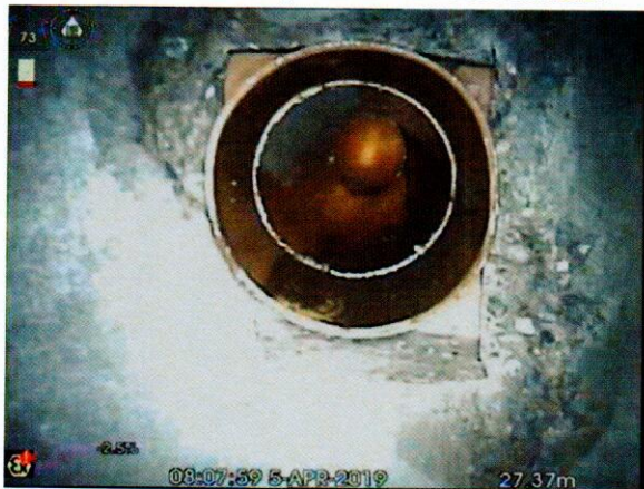
S5X_e997d85e-513a-4c9e-a330-d3a995be0e1e_20190405_090707_939.jpg, 00:04:08, 27.37 m Connection other than junction at 12 o'clock, diameter:
