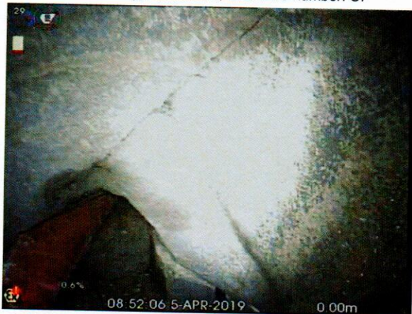
S7X_e95e40db-f421-4224-9e8c-5d1c64228623_20190405_095114_099.jpg, 00:00:24, 0.00 m Cracks, multiple from 4 o'clock to 6 o'clock
