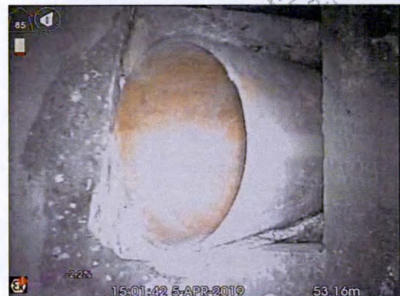
S11X_4159b65c-b355-45a4-92e8-229edce50242_20190405_160051_701.jpg, 00:08:06, 53.16 m Connection other than junction at 1 o'clock, diameter: 150mm
