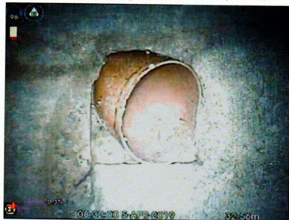
S6X_3f5f0a68-e51d-4e08-a22b-9b6fb0ced204_20190405_09 3108_985.jpg, 00:04:20, 32.56 m Connection other than junction at 12 o'clock, diameter:
