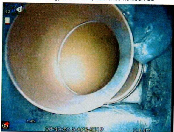
S5X_b7966323-76b6-459a-b1e1-98e9956461e4_20190405_094005_065.jpg, 00:00:28, 0.84 m Connection intruding at 2 o'clock, diameter: 100mm, intrusion:
