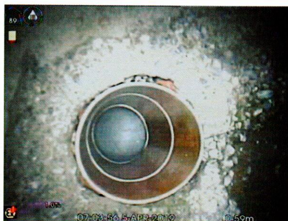
S4X_a5e9ed2b-8f8f-494b-b06d-fe2155b6fd24_20190405_080304_982.jpg, 00:00:11, 0.59 m Connection other than junction at 12 o'clock, diameter:
