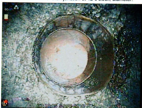
S4X_8113a11a-517e-4edd-8ac4-bde4a3698e20_20190405_080913_677.jpg, 00:04:43, 36.31 m Connection other than junction at 12 o'clock, diameter:
