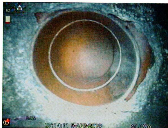
S4X_0a9403e3-fb40-4f72-b1bf-ef6ebd8fc1bf_20190405_081320_079.jpg, 00:08:11, 61.19 m Connection other than junction at 12 o'clock, diameter:
