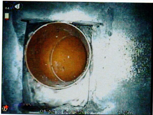
S5X_370e06e4-84f4-4c8a-a3a3-c44a2989c107_20190405_094118_654.jpg, 00:01:18, 4.75 m Connection other than junction at 1 o'clock, diameter: 100mm
