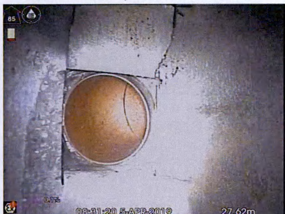
S6X_d6038f54-fdae-433f-a67f-0de6ba9aa6ba_20190405_093 028_351.jpg, 00:03:47, 27.62 m Connection other than junction at 12 o'clock, diameter:
