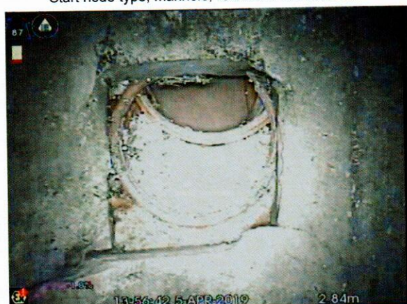
S12X_c8a29280-971f-4478-a52d-44cf951e9945_20190405_145551_027.jpg, 00:00:28, 2.84 m Connection other than junction at 12 o'clock, diameter:
