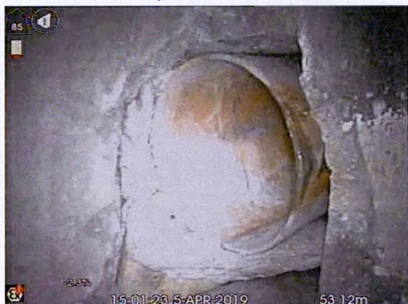
S11X_bced69d4-79c0-4d55-a302-6040b96b55cc_20190405_160032_561.jpg, 00:07:57, 53.11 m Connection other than junction at 1 o'clock, diameter: 150mm
