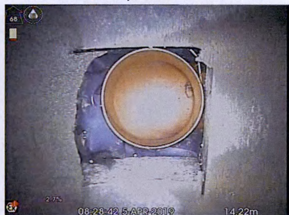
S6X_c9ec7afd-1a4f-4ea7-9098-e3660764c0f2_20190405_092750_886.jpg, 00:01:54, 14.22 m Connection other than junction at 12 o'clock, diameter:
