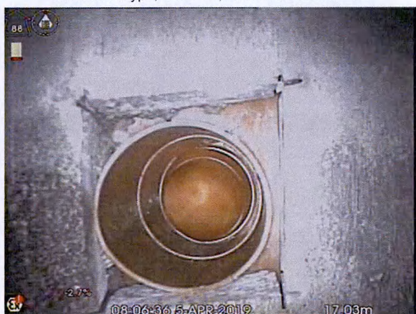
S5X_bd0ee04a-35e7-4a44-b67f-3794dc58536d_20190405_090545_028.jpg, 00:03:01, 17.03 m Connection other than junction at 12 o'clock, diameter:
