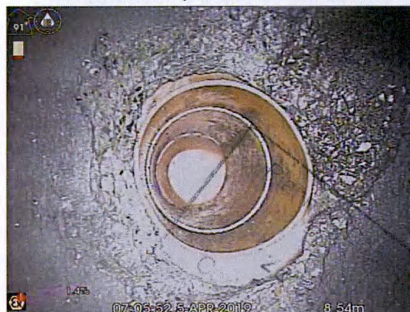
S4X_802735c8-86e0-42c0-8b8c-a67a50e5e5f3_20190405_08 80501_375.jpg, 00:01:12, 8.54 m Connection other than junction at 12 o'clock, diameter:
