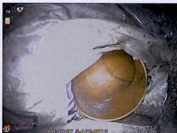
S5X_03b0457f-bb8e-468f-9713-1786b92e3fda_20190405_093935_556.jpg, 00:00:14, 0.42 m Connection other than junction at 2 o'clock, diameter: 100mm
