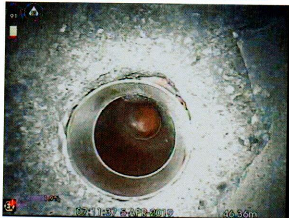
S4X_1c539c1b-af17-430a-a122-eb39745caf70_20190405_081045_894.jpg, 00:05:59, 46.36 m Connection other than junction at 12 o'clock, diameter:
