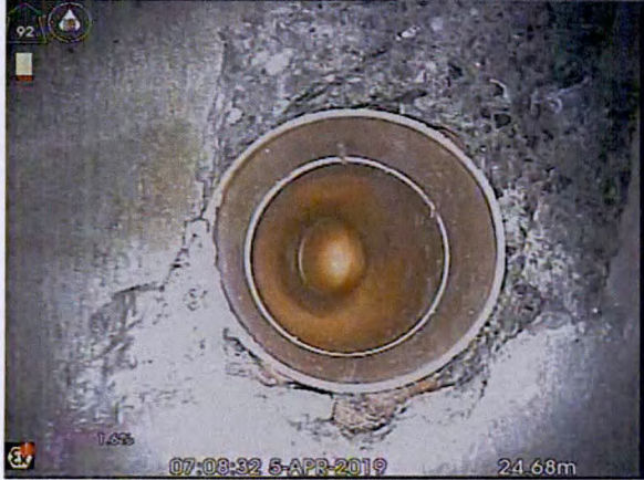
S4X_f6729a63-531b-46b9-9aaf-873fb425f930_20190405_080740_702.jpg, 00:03:25, 24.68 m Connection other than junction at 12 o'clock, diameter:
