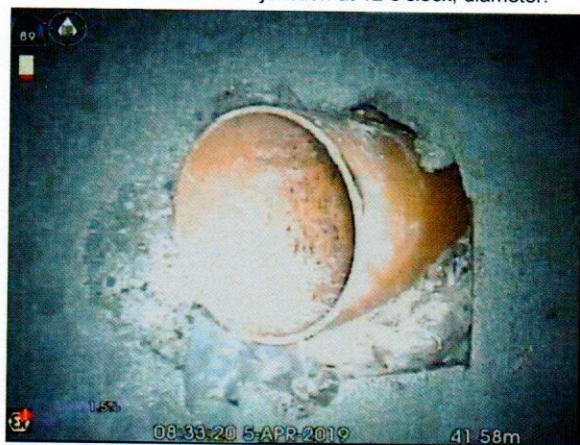
S6X_1735cf16-efdb-4b0a-88ca-38dbbd134ab1_20190405_09 3229_036.jpg, 00:05:23, 41.57 m Connection other than junction at 12 o'clock, diameter:
