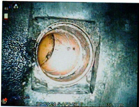
S5X_b30b547f-62c6-437a-8a7e-d78a072d496e_20190405_090834_506.jpg, 00:05:12, 36.11 m Connection other than junction at 12 o'clock, diameter:
