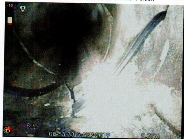
S7X_507b6eab-e483-4ccb-9798-b9840ae9fe90_20190405_095241_489.jpg, 00:01:01, 0.07 m Sealing ring broken from 3 o'clock to 9 o'clock
