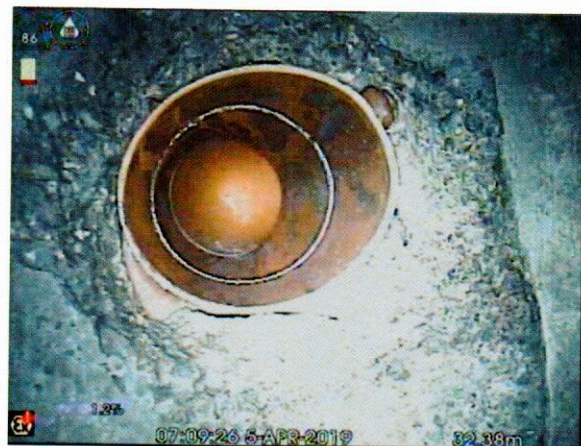
S4X_4dd6337d-9aba-4882-aa9d-5cf20b35e773_20190405_080834_359.jpg, 00:04:12, 32.38 m Connection other than junction at 12 o'clock, diameter:
