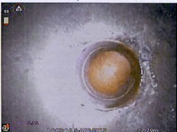
S12X_7c569883-7420-47af-be2e-602fc3a58e52_20190405_1 50225_562.jpg, 00:06:39, 27.79 m Connection other than junction at 12 o'clock, diameter:
