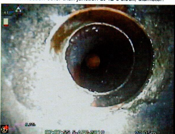
S4X_054fcaef-7066-4d99-b900-6afa1e02cb72_20190405_080704_434.jpg, 00:02:52, 22.05 m Connection other than junction at 12 o'clock, diameter:
