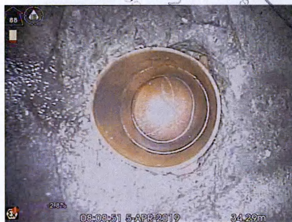
S5X_dc88f43e-10f2-439f-90a0-45b58179b8de_20190405_090759_213.jpg, 00:04:51, 34.29 m Connection other than junction at 12 o'clock, diameter:
