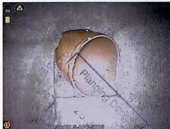
S6X_3f5f0a68-e51d-4e08-a22b-9b6f00ced204_20190405_09 3108_985.jpg, 00:04:26, 32.56 m Connection other than junction at 12 o'clock, diameter:
