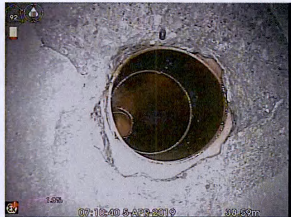
S4X_b34d13cd-a11f-4f5a-83bd-292a71613fec_20190405_080949_148.jpg, 00:05:11, 38.59 m Connection other than junction at 12 o'clock, diameter:
