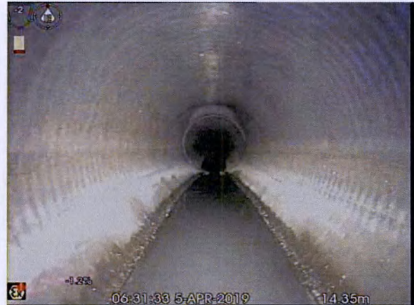
S2X_3c24dd86-e9c2-4854-a02e-26cc4f794fcc_20190405_073041_501.jpg, 00:01:20, 14.35 m Water level, 5% of the vertical dimension
