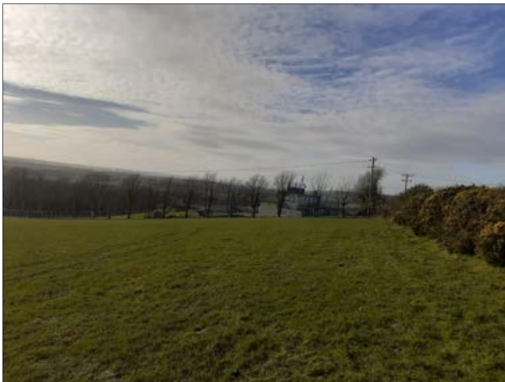
Plate 5. Water Treatment Plant, viewed from the east.
