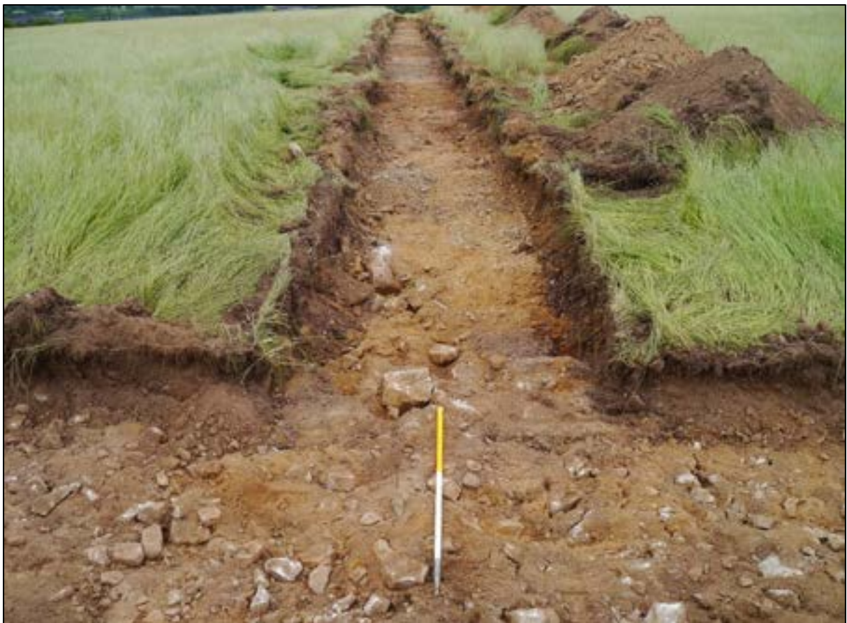
Plate 8: Trench 4 facing south-southeast
