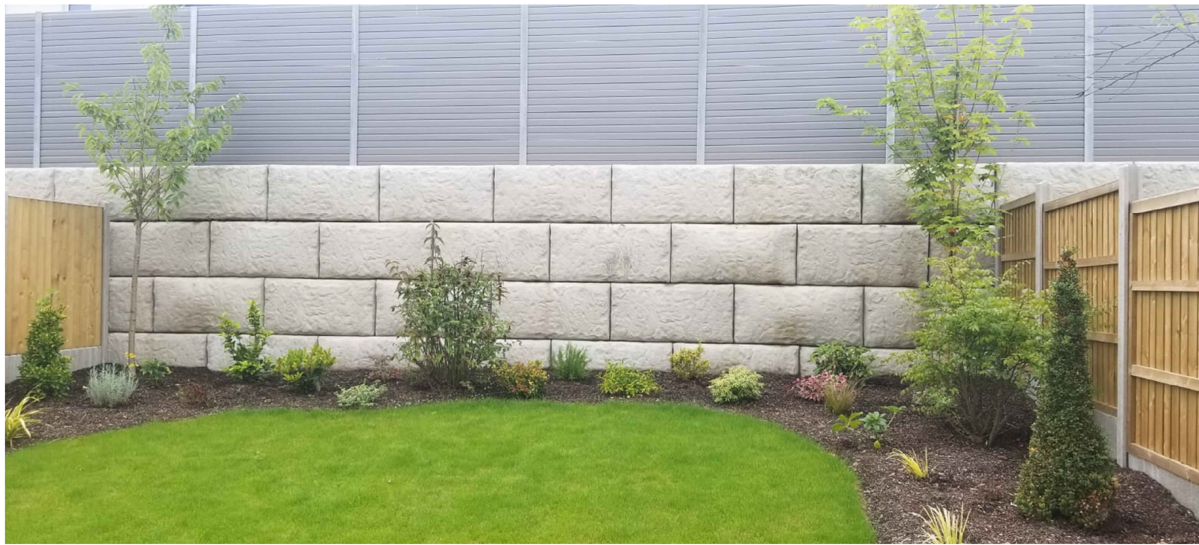
Example of Alfabloc retaining walls with concrete post & composit PVC paneling above including timber paneling between Houses
