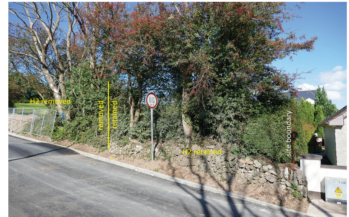
View from public road at southwest corner of site. Image illustrates the 10m segment of stone ditch and Hawthorn hedge to be retained at H2, plus diseased Elm and Ash trees to be removed and gap in ditch where there is no vegetation (also to be removed).
