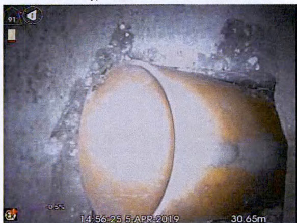
S11X_97e89ff1-cece-4ded-a60d-67b0788aebb6_20190405_155533_720.jpg, 00:03:15, 30.65 m Connection other than junction at 1 o'clock, diameter: 150mm
