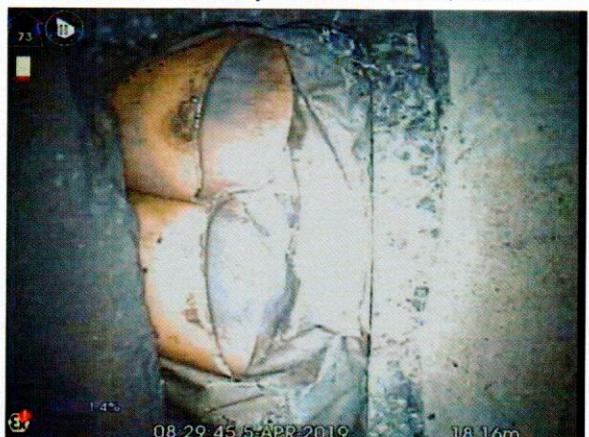
S6X_a74c1424-4840-47fc-b6ea-f90ae8ef89d6_20190405_092853_457.jpg, 00:02:37, 18.16 m Connection other than junction at 11 o'clock, diameter:
