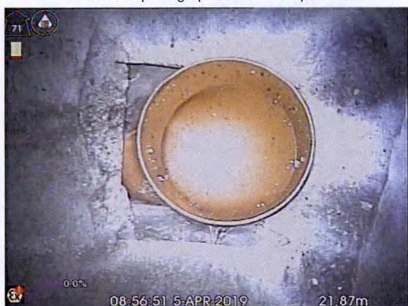
S7X_31436574-988a-4e7e-9a63-8803c35111fa_20190405_095559_947.jpg, 00:03:30, 21.87 m Connection other than junction at 12 o'clock, diameter:
