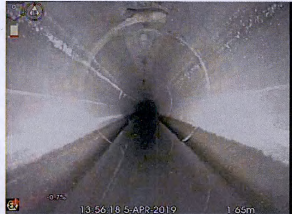
S12X_a4c78e13-8fa1-48da-99c7-0acaecf3be4c_20190405_1 45527_027.jpg, 00:00:12, 1.65 m Water level, 10% of the vertical dimension
