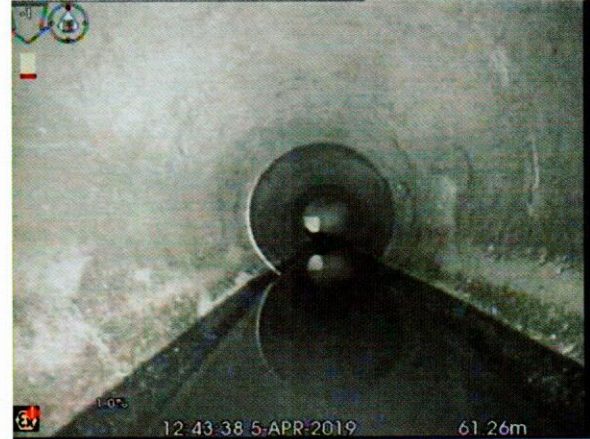
S10X_f3b594ef-ef55-4d79-baf5-181129d52886_20190405_13 4246_959.jpg, 00:05:21, 61.26 m Water level, 10% of the vertical dimension
