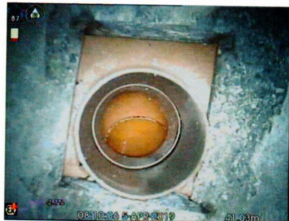
S5X_a2af812d-00a0-49d5-82f5-9c2578d3b00a_20190405_090914_929.jpg, 00:05:45, 41.03 m Connection other than junction at 12 o'clock, diameter:
