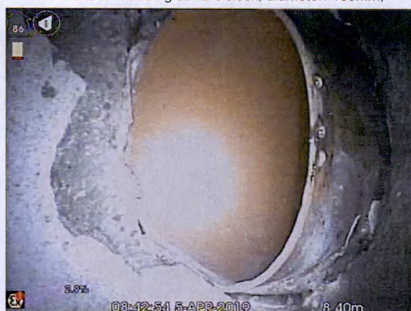
S5X_acceb949-f9b9-48f2-85ef-1e599e766fc5_20190405_094202_125.jpg, 00:01:52, 8.40 m Connection other than junction at 2 o'clock, diameter: 100mm
