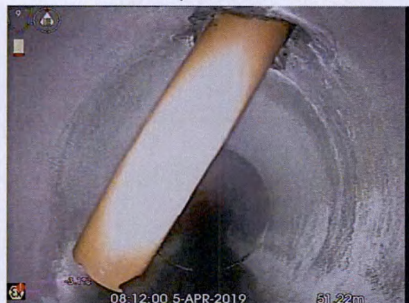
S5X_d9c04386-cfdb-4432-a2e0-6620da3a2084_20190405_091108_192.jpg, 00:06:56, 51.22 m Connection intruding at 1 o'clock, diameter: 100mm, intrusion:
