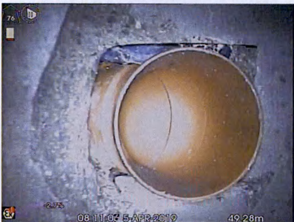
S5X_5188388e-7b81-4df1-9aaa-194757a45e84_20190405_091014_963.jpg, 00:06:34, 49.28 m Connection other than junction at 11 o'clock, diameter:
