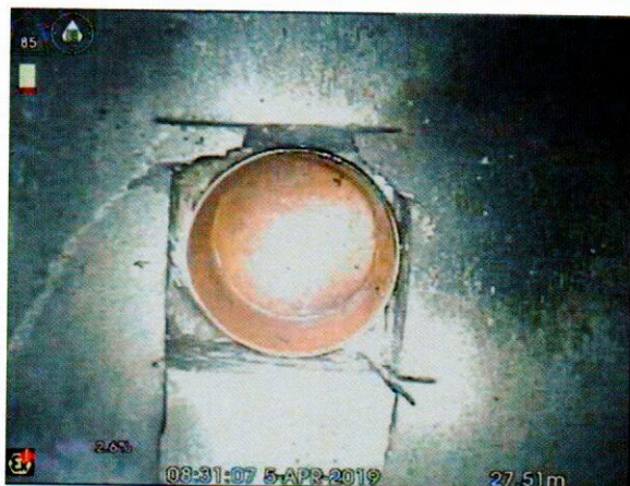
S6X_906c9892-9f70-4388-9326-8bfcfe449905_20190405_09 3015_084.jpg, 00:03:41, 27.51 m Connection other than junction at 12 o'clock, diameter:
