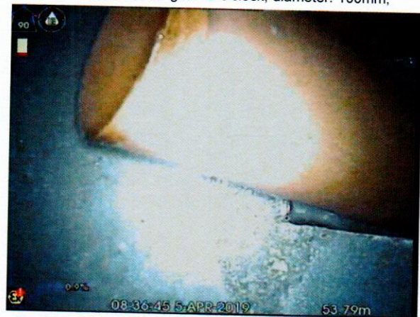
S6X_db2ccba5-02ab-4808-a2f3-f6fb28bc5a34_20190405_093553_252.jpg, 00:07:32, 53.79 m Connection intruding at 12 o'clock, diameter: 100mm,
