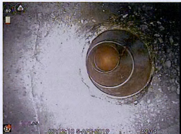
S4X_70a28ef5-6797-4dd6-b806-d4c54aea946f_20190405_081119_111.jpg, 00:06:25, 49.34 m Connection other than junction at 12 o'clock, diameter:
