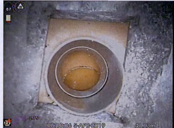
S5X_a2af812d-00a0-49d5-82f5-9c2578d3b00a_20190405_090914_929.jpg, 00:05:45, 41.03 m Connection other than junction at 12 o'clock, diameter:
