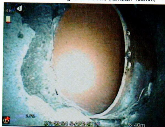
S5X_acceb949-f9b9-48f2-85ef-1e599e766fc5_20190405_094202_125.jpg, 00:01:52, 8.40 m Connection other than junction at 2 o'clock, diameter: 100mm
