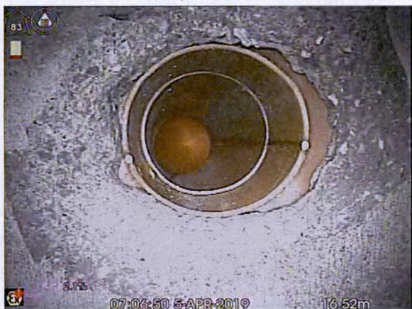
S4X_0a309ee2-7cfd-4233-bd52-868781fad4a2_20190405_08 0558_786.jpg, 00:02:01, 16.53 m Connection other than junction at 12 o'clock, diameter:
