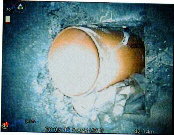
S6X_28decd9d-07d9-44c7-92b2-5de24c9dc43b_20190405_093250_338.jpg, 00:05:35, 42.14 m Connection other than junction at 12 o'clock, diameter:
