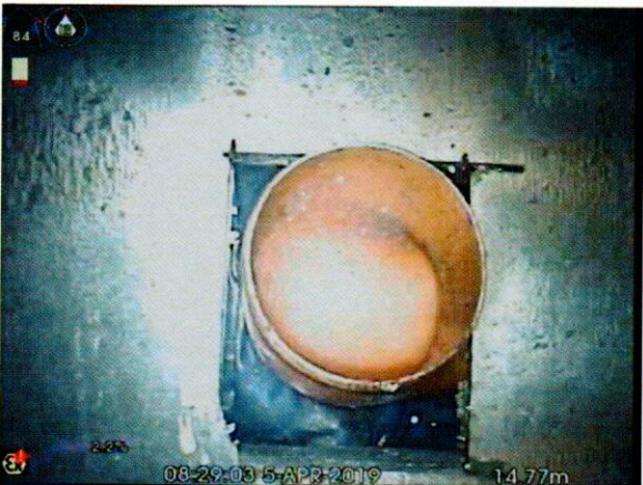
S6X_81383c55-9e7a-4746-8099-ef1c849ac6b8_20190405_092812_269.jpg, 00:02:07, 14.77 m Connection other than junction at 12 o'clock, diameter:
