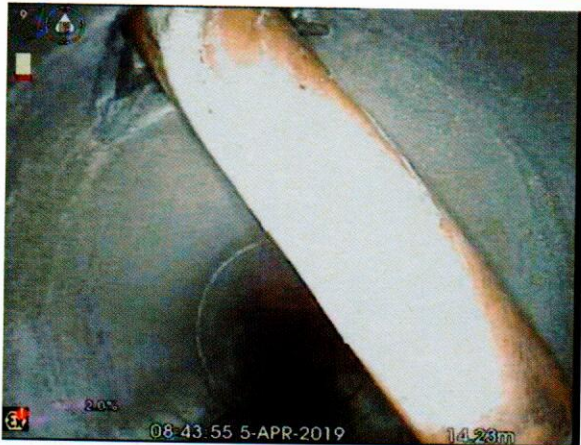
S5X_1b0d48cc-b4e9-416a-a0f1-9fd0bb0d32b9_20190405_094303_328.jpg, 00:02:36, 14.23 m Connection intruding at 11 o'clock, diameter: 100mm,
