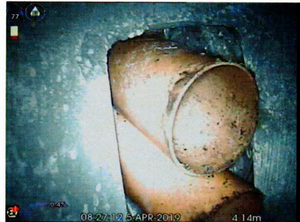
S6X_91b31115-cf97-4745-8a43-0827462e78b0_20190405_092621_053.jpg, 00:00:39, 4.14 m Connection other than junction at 12 o'clock, diameter:
