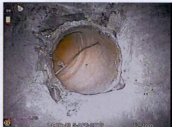
S12X_1bd62a68-ad66-4de4-b315-8e019f14ab10_20190405_1 145952_710.jpg, 00:04:18, 12.36 m Connection other than junction at 12 o'clock, diameter:
