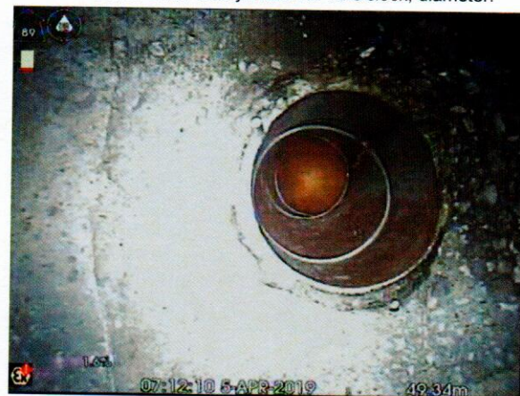
S4X_70a28ef5-6797-4dd6-b806-d4c54aea946f_20190405_081119_111.jpg, 00:06:25, 49.34 m Connection other than junction at 12 o'clock, diameter:
