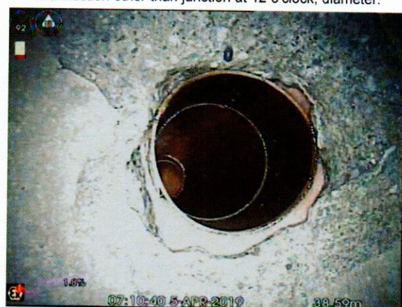
S4X_b34d13cd-a11f-4f5a-83bd-292a71613fec_20190405_080949_148.jpg, 00:05:11, 38.59 m Connection other than junction at 12 o'clock, diameter:
