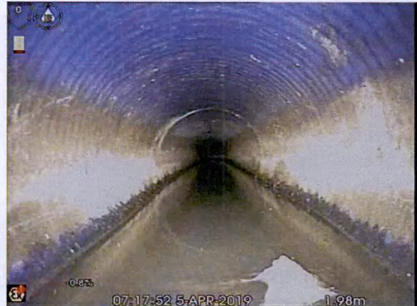
S3X_51ac9785-3074-40fa-9406-ab5ca25e2d2c_20190405_0 81701_604.jpg, 00:00:51, 1.98 m Water level, 20% of the vertical dimension
