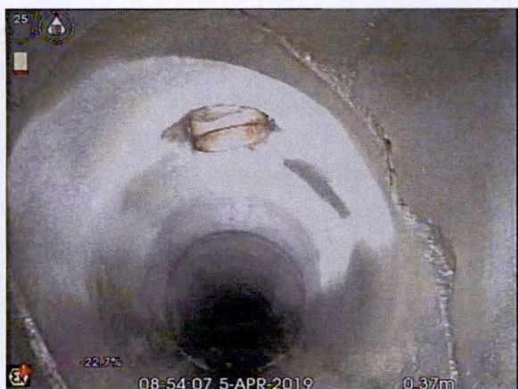
S7X_7668e268-54dd-4054-bff4-0173f5f9763b_20190405_095314_961.jpg, 00:01:21, 0.37 m Cracks, spiral from 12 o'clock to 12 o'clock
