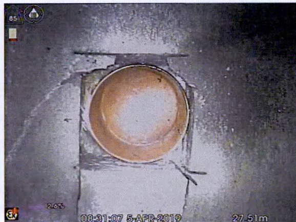
S6X_906c9892-9f70-4388-9326-8bfcfe449905_20190405_09 3015_084.jpg, 00:03:41, 27.51 m Connection other than junction at 12 o'clock, diameter:
