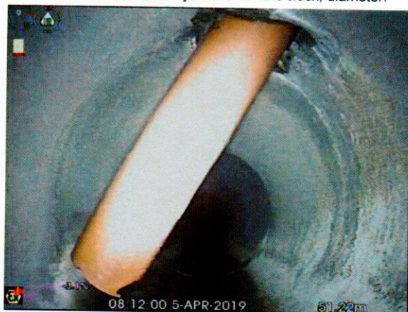
S5X_d9c04386-cfdb-4432-a2e0-6620da3a2084_20190405_091108_192.jpg, 00:06:56, 51.22 m Connection intruding at 1 o'clock, diameter: 100mm, intrusion:
