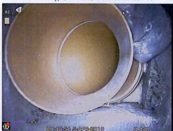
S5X_b7966323-76b6-459a-b1e1-98e9956461e4_20190405_094005_065.jpg, 00:00:28, 0.84 m Connection intruding at 2 o'clock, diameter: 100mm, intrusion:
