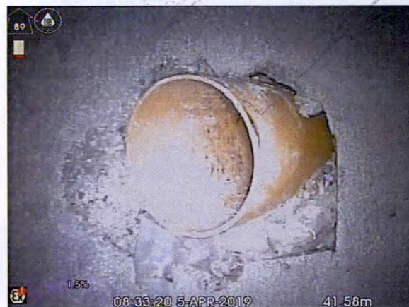
S6X_1735cf16-efdb-4b0a-88ca-38dbbd134ab1_20190405_09 3229_036.jpg, 00:05:23, 41.57 m Connection other than junction at 12 o'clock, diameter:
