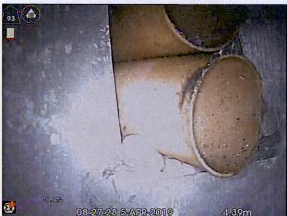
S6X_a4098aa4-0653-4636-a51a-36339279b92e_20190405_092636_205.jpg, 00:00:46, 4.39 m Connection other than junction at 12 o'clock, diameter:
