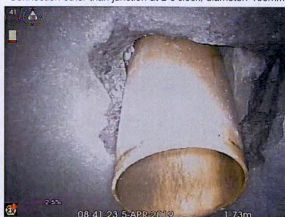
S5X_62aa0cc2-107c-47cd-adfc-3f77a6d3f8cb_20190405_094031_971.jpg, 00:00:43, 1.73 m Connection intruding at 12 o'clock, diameter: 100mm,
