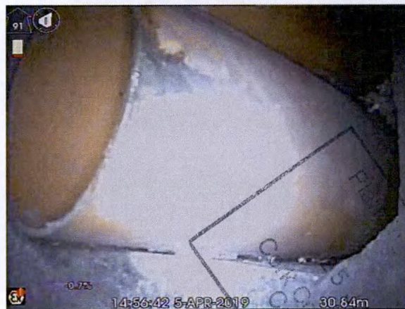
S11X_b51732fa-f87c-498b-98f5-c59dd0c10ad3_20190405_155550_998.jpg, 00:03:25, 30.64 m Connection other than junction at 1 o'clock, diameter: 150mm
