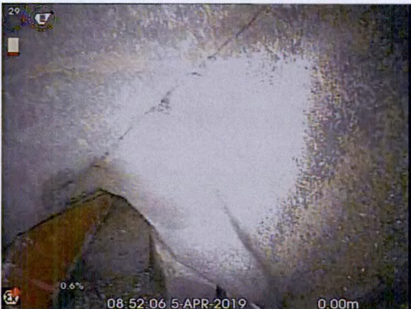
S7X_e95e40db-f421-4224-9e8c-5d1c64228623_20190405_095114_099.jpg, 00:00:24, 0.00 m Cracks, multiple from 4 o'clock to 6 o'clock
