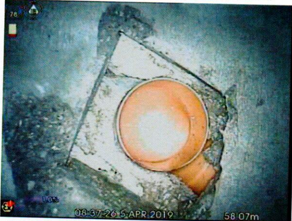
S6X_c5a221d9-8216-4a70-82c9-317fa8dbc8cf_20190405_093635_123.jpg, 00:08:05, 58.07 m Connection other than junction at 12 o'clock, diameter:
