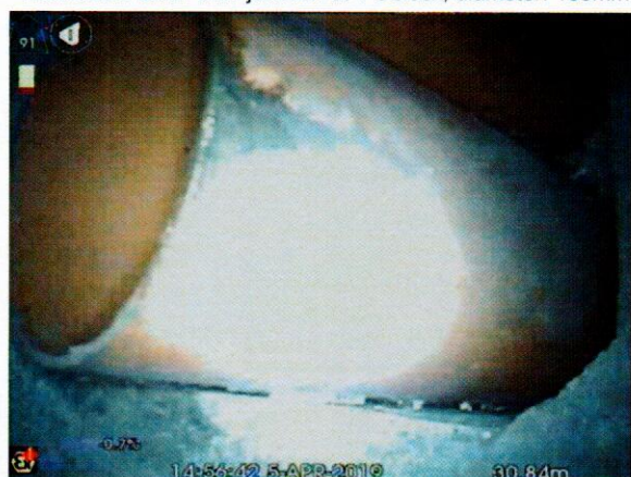
S11X_b51732fa-f87c-498b-98f5-c59dd0c10ad3_20190405_155550_998.jpg, 00:03:25, 30.84 m Connection other than junction at 1 o'clock, diameter: 150mm
