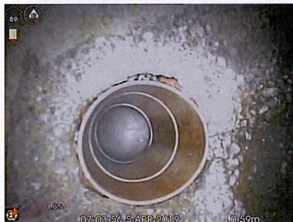
S4X_a5e9ed2b-8f8f-494b-b06d-fe2155b6fd24_20190405_08 304_982.jpg, 00:00:11, 0.59 m Connection other than junction at 12 o'clock, diameter:
