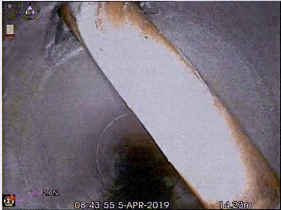
S5X_1b0d48cc-b4e9-416a-a0f1-9fd0bb0d32b9_20190405_094303_328.jpg, 00:02:36, 14.23 m Connection intruding at 11 o'clock, diameter: 100mm,
