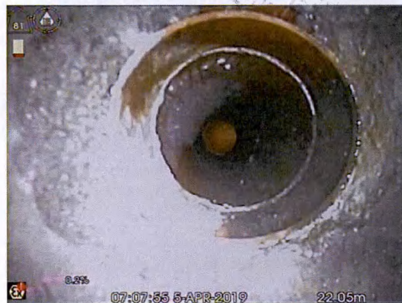
S4X_054fcaef-7066-4d99-b900-6afa1e02cb72_20190405_08 0704_434.jpg, 00:02:52, 22.05 m Connection other than junction at 12 o'clock, diameter:
