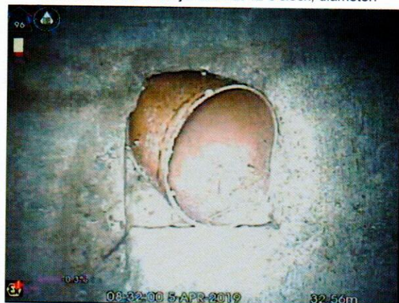
S6X_3f5f0a68-e51d-4e08-a22b-9b6fb0ced204_20190405_09 3108_985.jpg, 00:04:20, 32.56 m Connection other than junction at 12 o'clock, diameter:
